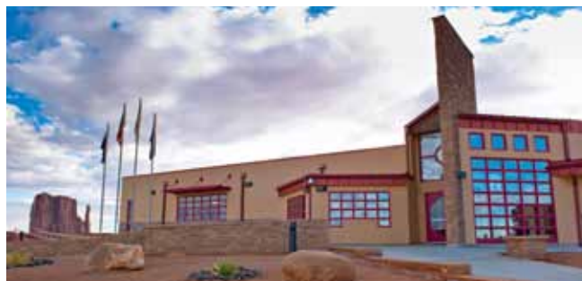
The recently completed visitor center project at Monument Valley Navajo Tribal Park
